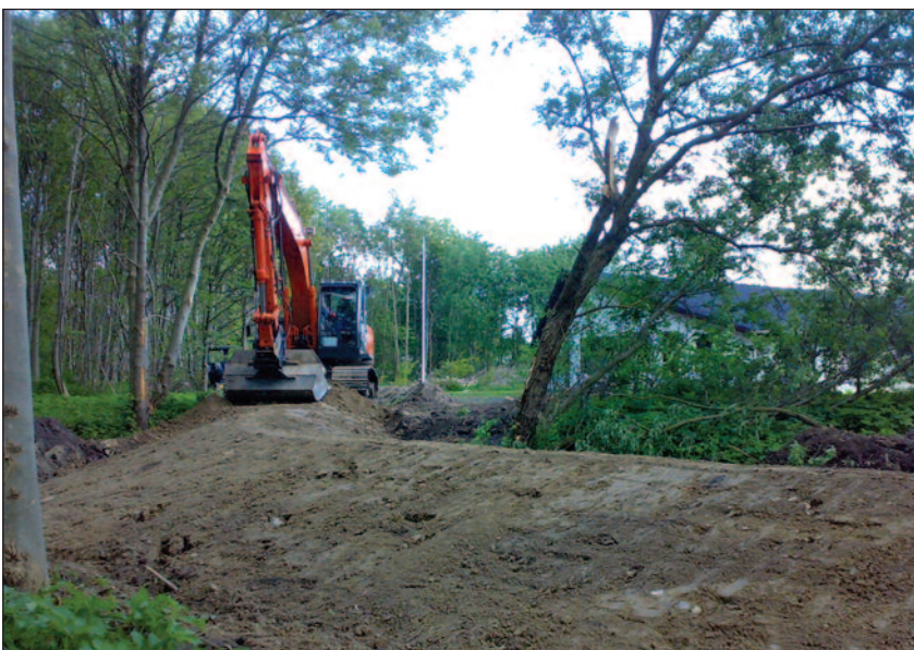
Example of adaption measures in Greve. A new barrier is being built to prevent future flooding. Photo: Greve municipality.
